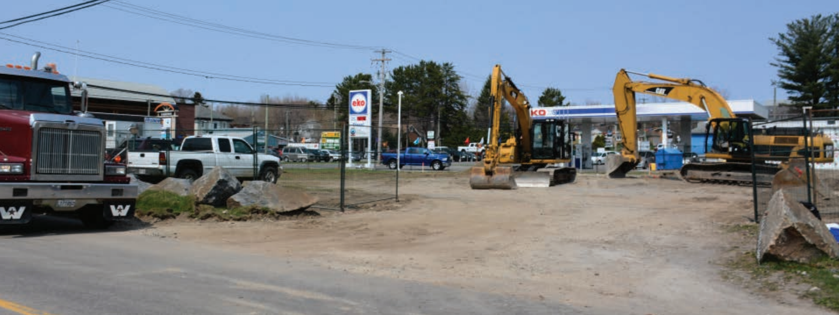
Construction is underway Photo : Mélanie Vincent
